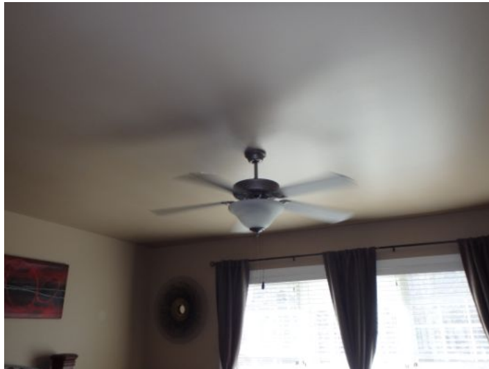
Ceiling fan in the master bedroom wobbles. May need a balance kit installed.
