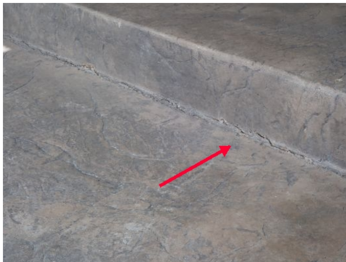
Cracking that has occurred due to settlement of the front porch.
