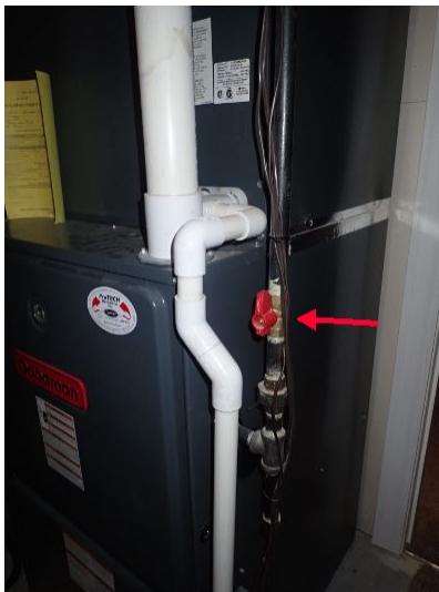
Furnace gas cut off valve
