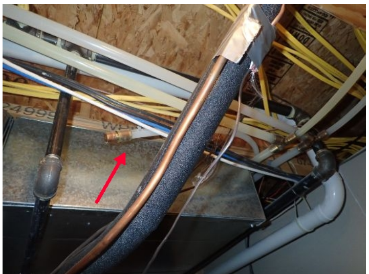
DEDICATED LOOP HOT WATER RECIRCULATION SYSTEM
