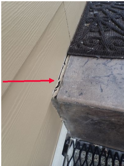
Separation between house wall and porch at the north side of the home.
