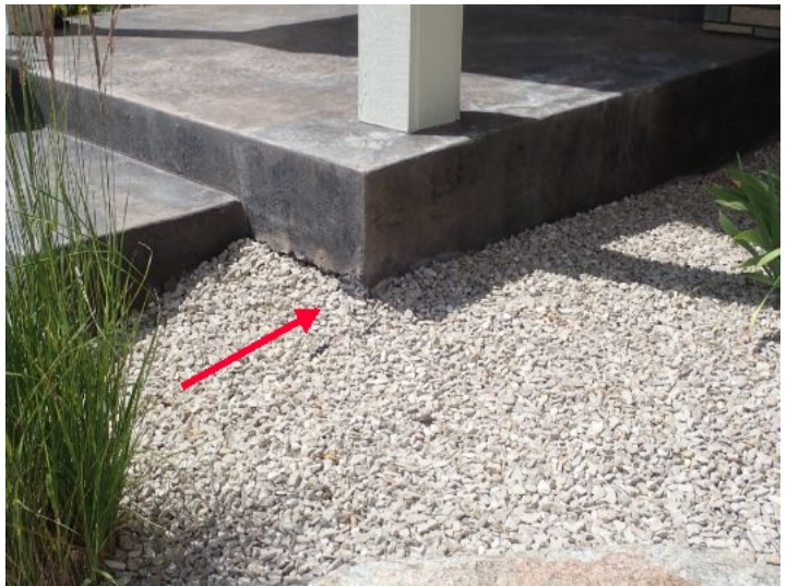
Note the lack of supporting soils under this corner of the concrete front porch.
